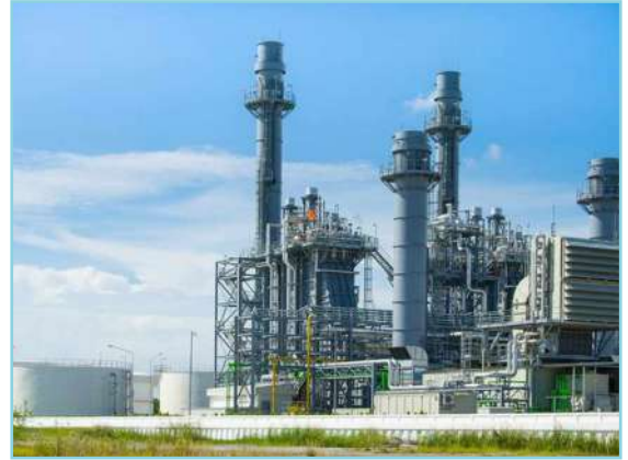
Installation of PVC pipes & fittings for Chlorine Dosing System at Shuwaikh Power Plant (Client: Doosan Engineering Co – Korea)
