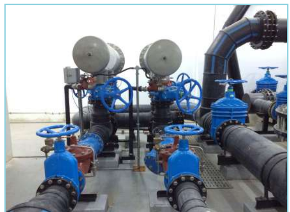
Supply & Installation of HDPE & PVC pipes and fittings
