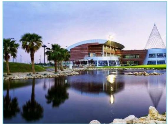
Installation of large HDPE pipe (Dia 315mm) & fittings Sahara Golf Club, Kuwait
