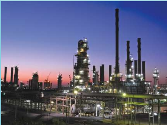
Supply & installation of HDPE gravity pipes and fittings KNPC Mina Abdullah Refinery, Ammonia Injection CB/1259
