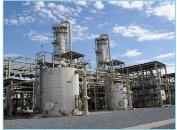
Joint Operations (Chevron) at Wafra Installation of HDPE pipeline (Client: Gulf Combined Est. – KSA)
