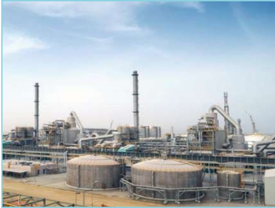
Repair and Upgrading piping systems Bulk Acid Plant. Ahmadi, Kuwait (Client: Haliburton Overseas Ltd.)
