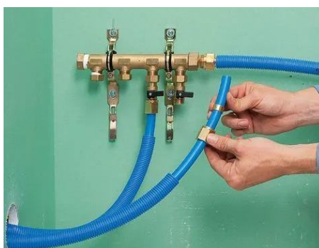
Compression Fittings Manifold Installation
