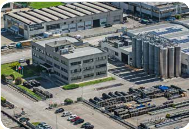
Production and Operations Centre - Castel Guelfo di Bologna (BO) - Italy
