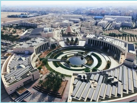
HDPE external work & Firefighting piping system PAAET Project Student Campus at Ardiya (M/s. United Gulf Construction Co. – UGCC)
