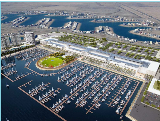
Installation of MEP works, Laying of electrical cables and HDPE pipes & fittings for pontoons on Marina Jetty Sabah Al Ahmad Sea City Phase A2
