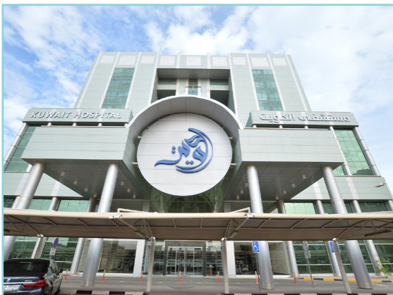
Installation of HDPE works for pump room Mubarak Hospital (Client: Ali Alghanim & Sons)
