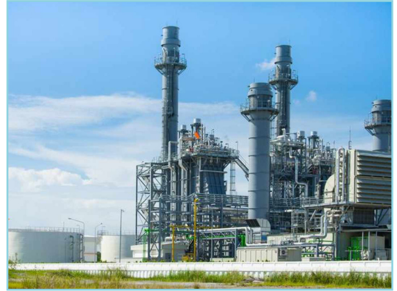
Installation of PVC pipes & fittings for Chlorine Dosing System at Shuwaikh Power Plant (Client: Doosan Engineering Co – Korea)
