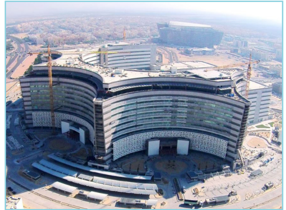
Design, Supply, Installation and Maintenance of Temporary firefighting system consisting of HDPE underground pipes and above ground steel pipes Jaber Al Ahmad Al Jaber Al Sabah Hospital
