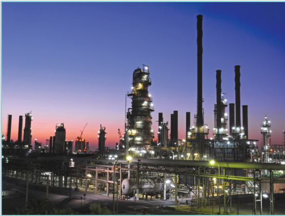
Supply & installation of HDPE gravity pipes and fittings KNPC Mina Abdullah Refinery, Ammonia Injection CB/1259
