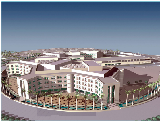
Installation of HDPE pipes & Fittings Kuwait Oil Company, Ahmadi (Client: Turki Al Dabbos)
